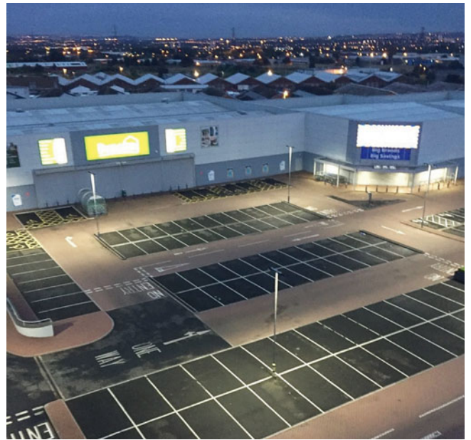
External car park lighting replacement programme at North Shields, completed in August 2016.
